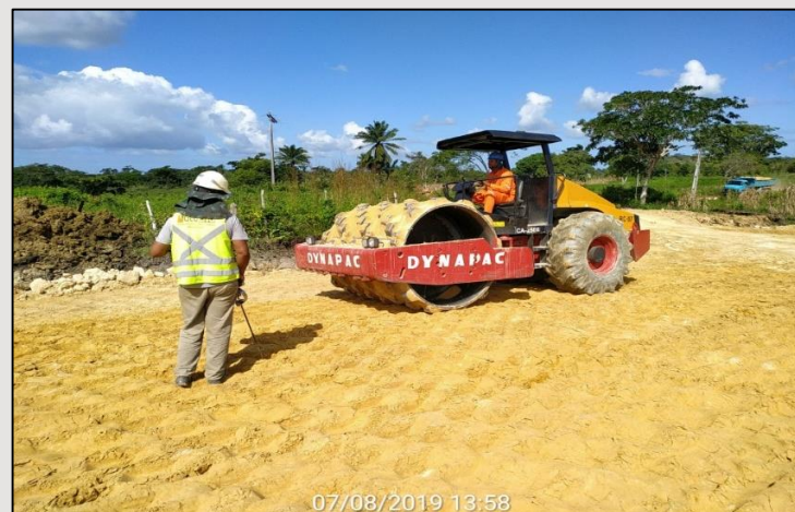
UGN Site Compaction
